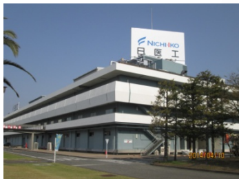
Nichi-Iko Pharma Tech Shizuoka Plant
